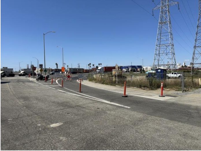
On-Ramp to S/B SR-103 from I Street
